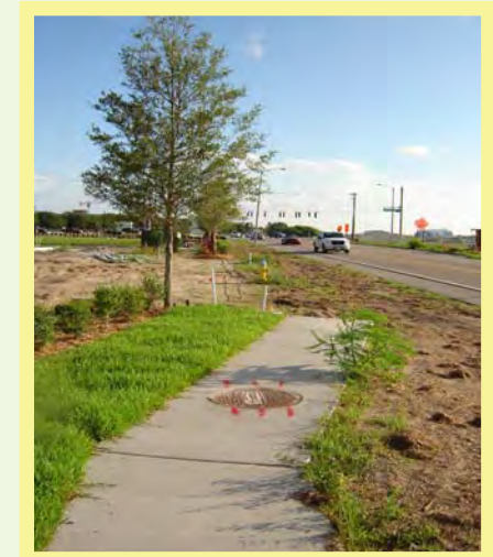
New Sidewalk on O'Brien Street
