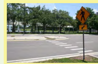
Continental crosswalk pattern on George Road
