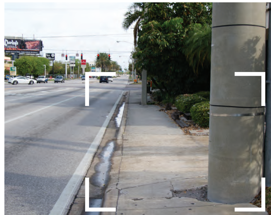
Constrained Sidewalk Width- Placement of Infrastructure Features
