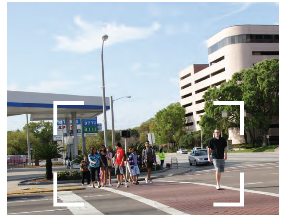
Wide Crosswalk Width Limiting Safe Pedestrian Crossing
