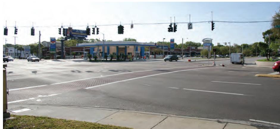
Existing Intersection Conditions at Westshore Boulevard and Kennedy Boulevard
