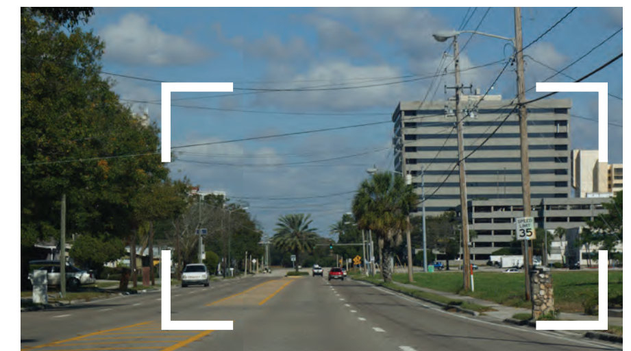
Existing Conditions Along Lois Avenue-Looking North
