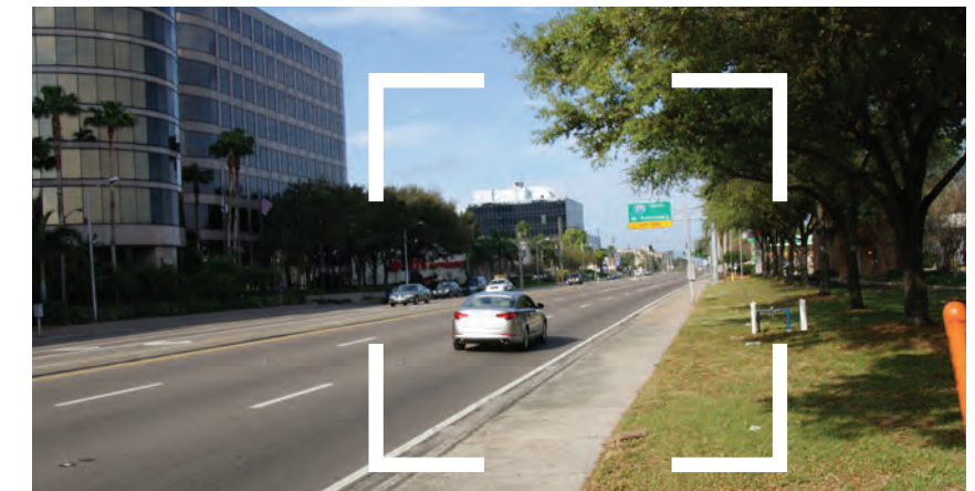
Existing Sidewalk Conditions along Kennedy Boulevard
