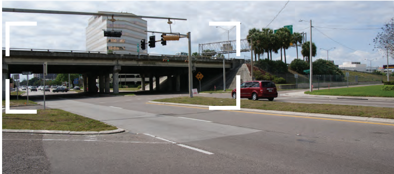
Existing Public Real Conditions at I-275/Westshore Boulevard Bridge Underpass
