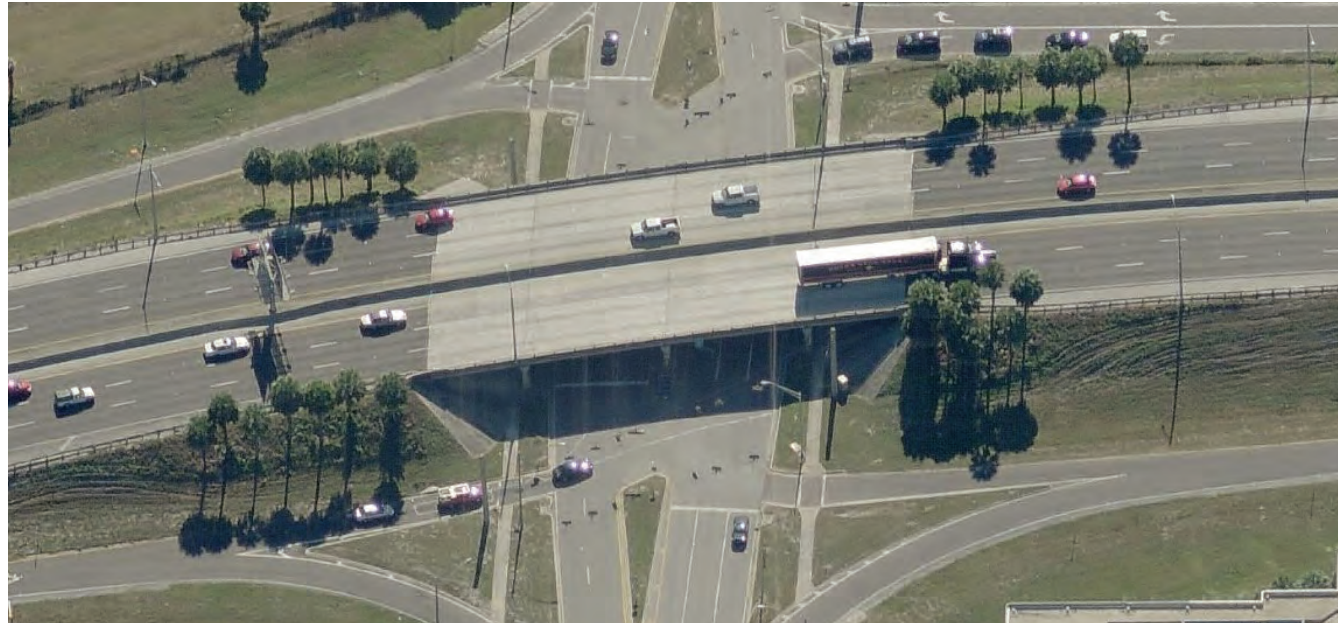
Existing Public Real Conditions at Lois Avenue/I-275 Bridge Overpass
