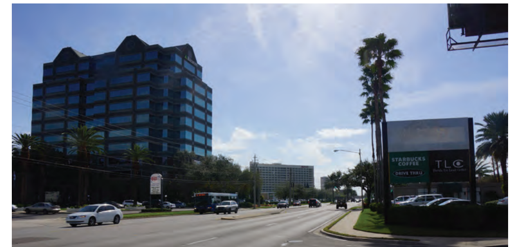
Existing Conditions Along Westshore Boulevard Looking South
