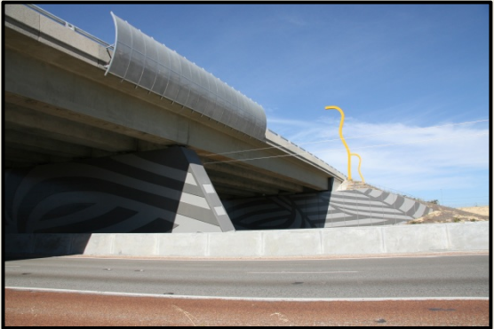
REPRESENTATIVE VIADUCT PORTAL/ABUTMENT WALL FEATURES
