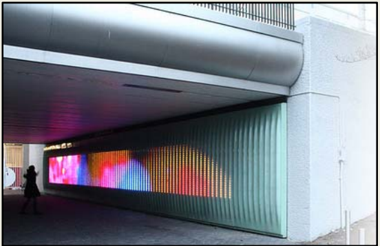
REPRESENTATIVE VIADUCT PORTAL/ABUTMENT WALL FEATURES
