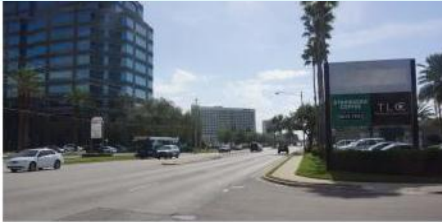
EXISTING CONDITION ON WESTSHORE BOULEVARD
