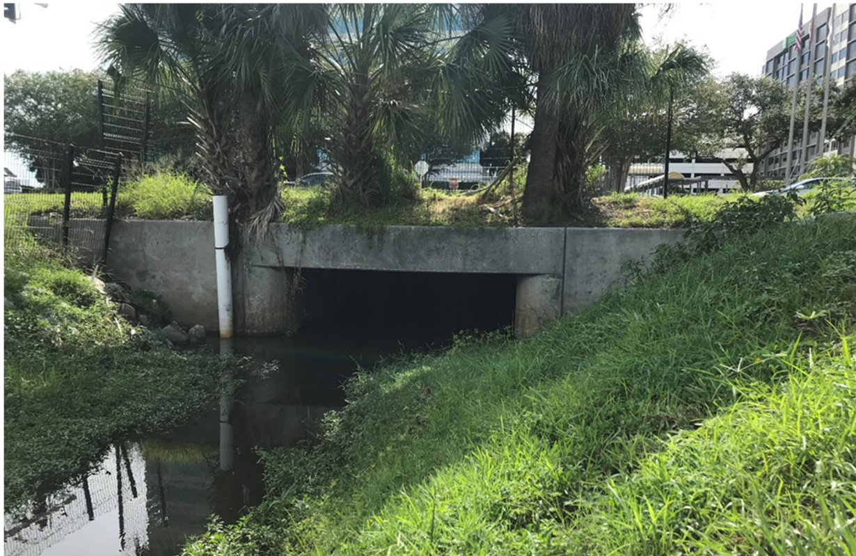
Figure 2-16: Lemon Street Box Culvert
