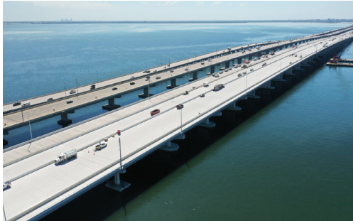
HOWARD FRANKLAND BRIDGE I-275 8 Lanes (4 General Use & 4 Express)
