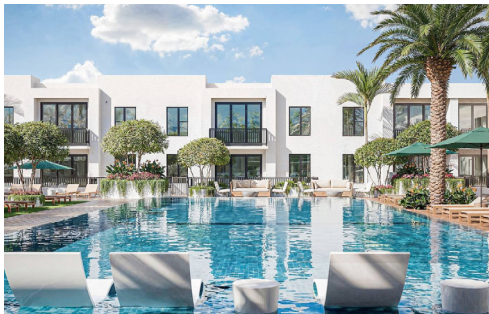
THE EMERALD AT METWEST 8-Story 375 Units
