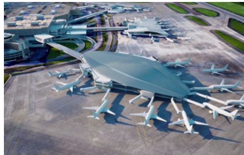
TAMPA INTERNATIONAL AIRPORT AIRSIDE D
